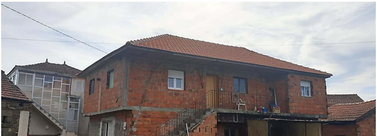
Roof Rehabilitation at a house at Covas do Barroso
