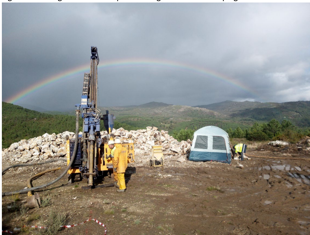
Figure 1: Drilling at the NOA deposit during the current campaign
