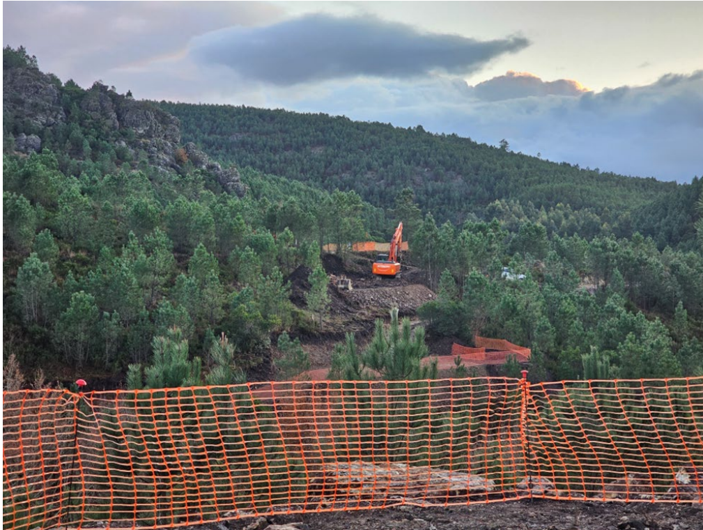
Figure 1: Drill pad preparation underway at the Pinheiro deposit
